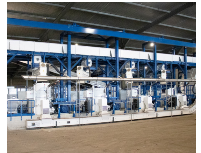
↑ Recycling plant with a throughput of 85,000 t/a
