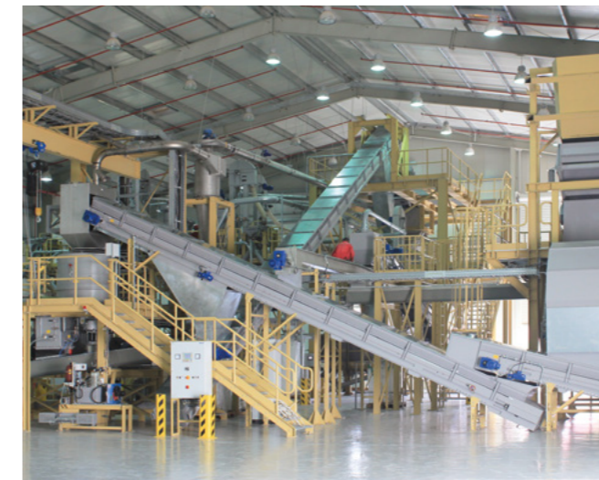
↑ Recycling plant with a throughput of 20,000 t/a
